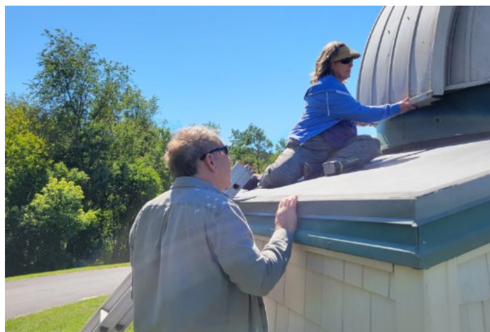
Laurie & Al work to seal the observatory dome
